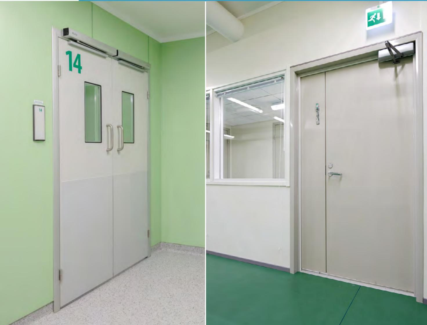
The fastening of the closer and opening device is carried out using 3 mm thick steel plate in the middle of the door leaf. The width and height are in accordance with the type of chosen device.
