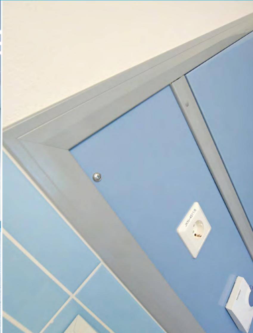
Side panels can accommodate switches, controls etc – items which are normally wall fixed
